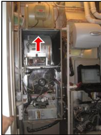
J. Picture 1 Arrow shows area where water came from
